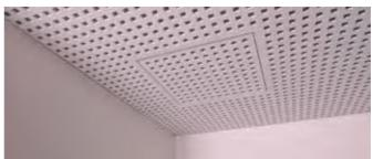
The factory-integrated perforated panel lid ensures a homogeneous integration into the ceiling surface with a frieze area that is not or only minimally non-perforated, depending on the perforation pattern. (Exception: random perforation panels should always be fitted into place at the job site)
